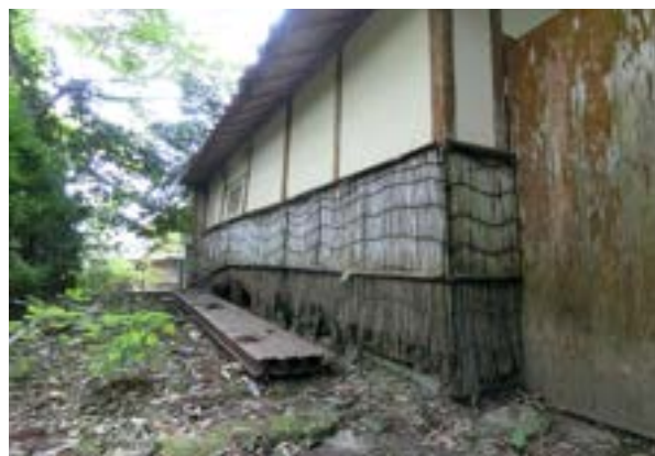
図3-1-30 物置の腐朽
