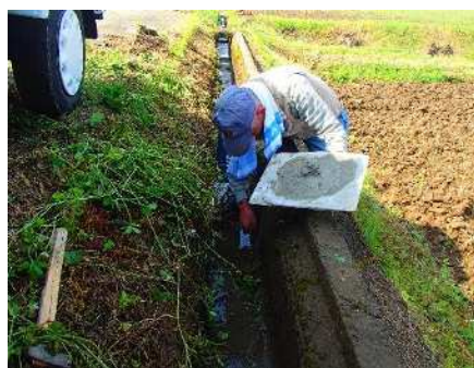
[水路の目地詰め]
