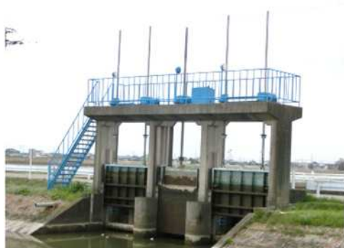
[制水門補修前]
