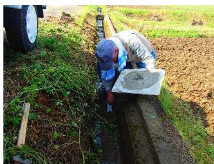
[水路の目地詰め]
